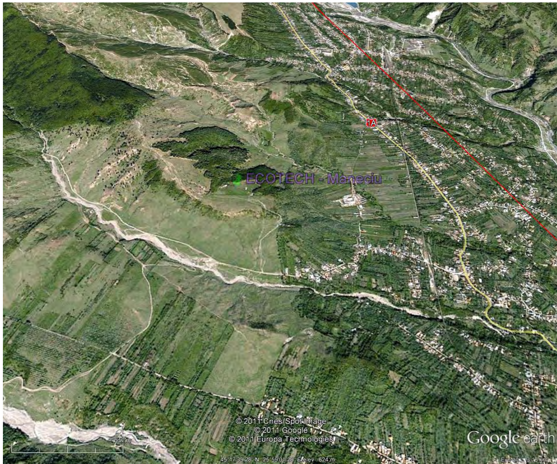
INCAS location on Maneciu Platform - (11 ha, 2.800m 2 offices)
